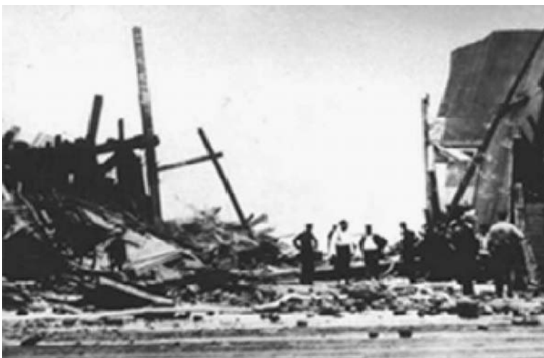
Debris from the explosion.
