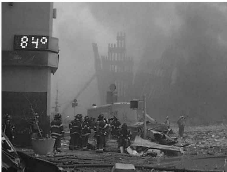
Dust covered street.
