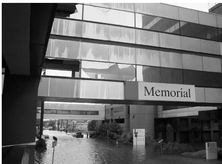
Damaged crosswalk at Baptist Hospital; street flooding below.
